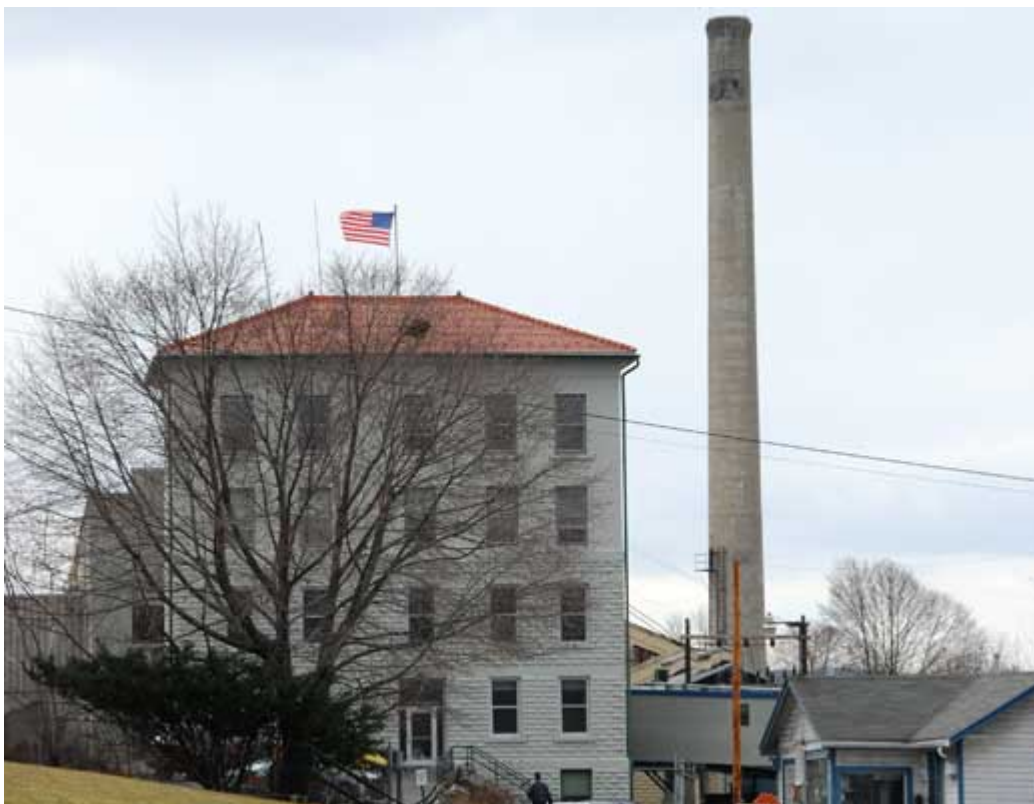
A view of Emerson Power Transmission buildings from the company parking lot. The company's location is the site of pollution from its former tenant, Morse Industrial, that the DEC is attempting to clean up. (Photo by Rachel Philipson)
